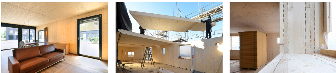
Woodcube is designed by a German architectural office, Architekturgentur, in 2013. It is based on Holz100 -massive wood elements that are totally glueless as well as metal and plastic free. Source: Arch Daily, Pictures: Martin Kunze
