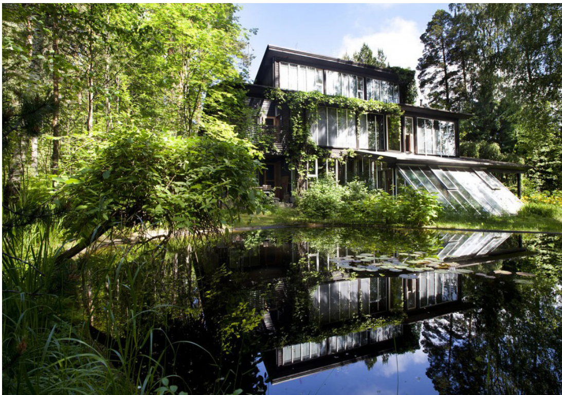
Villa Solbrante's windows face mainly south and the house uses passive and active solar energy for general heating and heating the service water. Picture: Bruno Erat.
