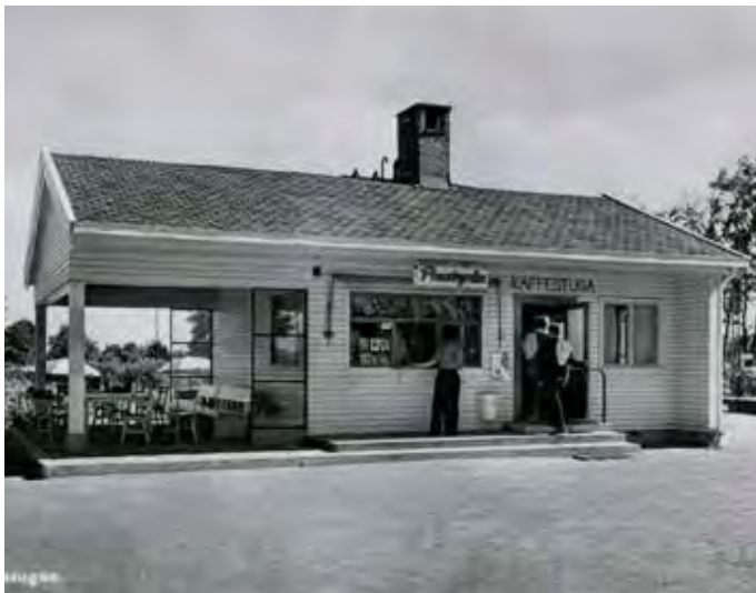
Kiosk and café where the new station building is now [7]
