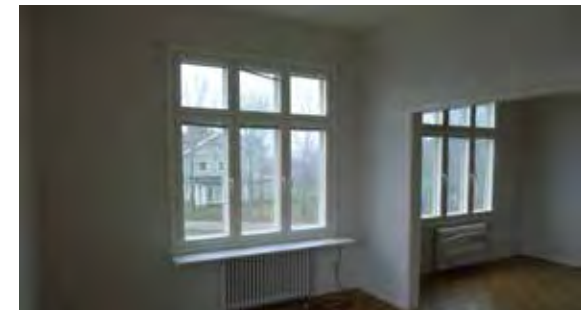
Large windows in the future office spaces
