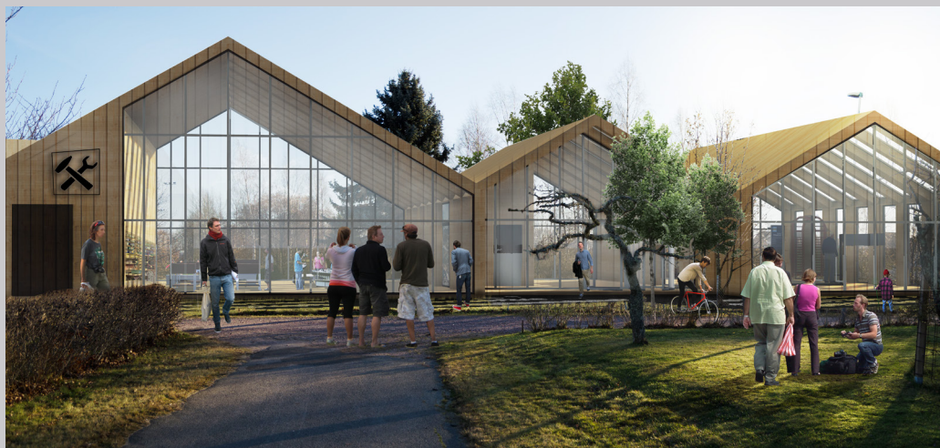
View of the exhibition and workshop building from West
