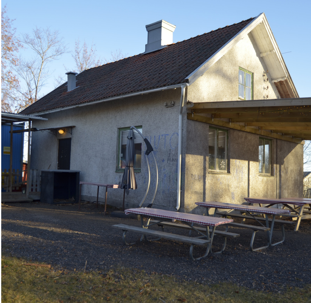
Existing building on the site
