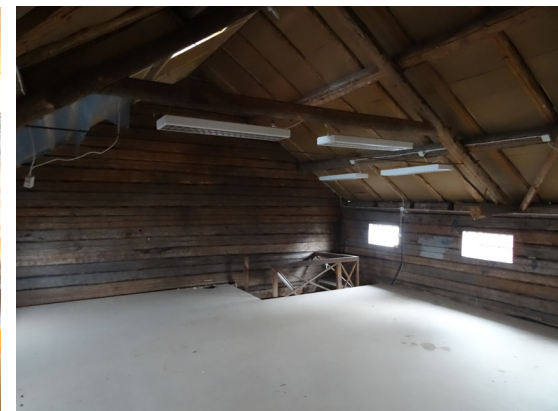
The first floor was not used when the building was a restaurant. It is also non-insulated.
