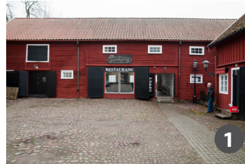
"Grönköping" - a two storey building build in timber from before 1837. Original it was used for storage and as barn, but during the lastest years, until 2016, it has been used as a restaurant and café.
