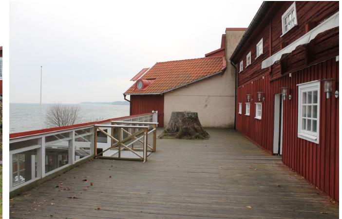
Between the building and the two rooms. It also has great views to the Lake.
