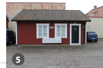
One storey building from the 1980's, used as a workshop for leather handicraft.
