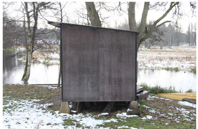
The shed is a marvel in pragmatism and common sense. It rests on concrete pylons rather than slabs, so it touches the earth lightly. Its roof cantilevers when necessary.
