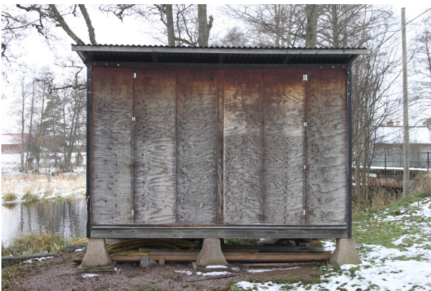
The shed is a marvel in pragmatism and common sense. It rests on concrete pylons rather than slabs, so it touches the earth lightly. Its roof cantilevers when necessary.
